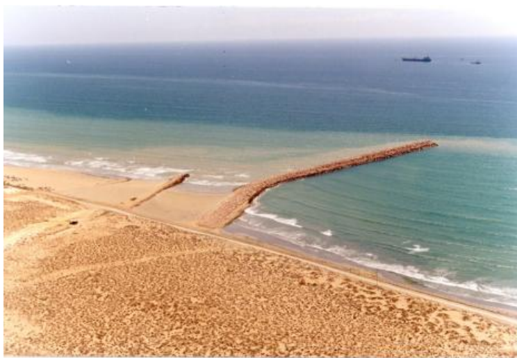
Figure 2-1: Longshore Sediment Transport around a Groyne (Drift Direction from L to R)
