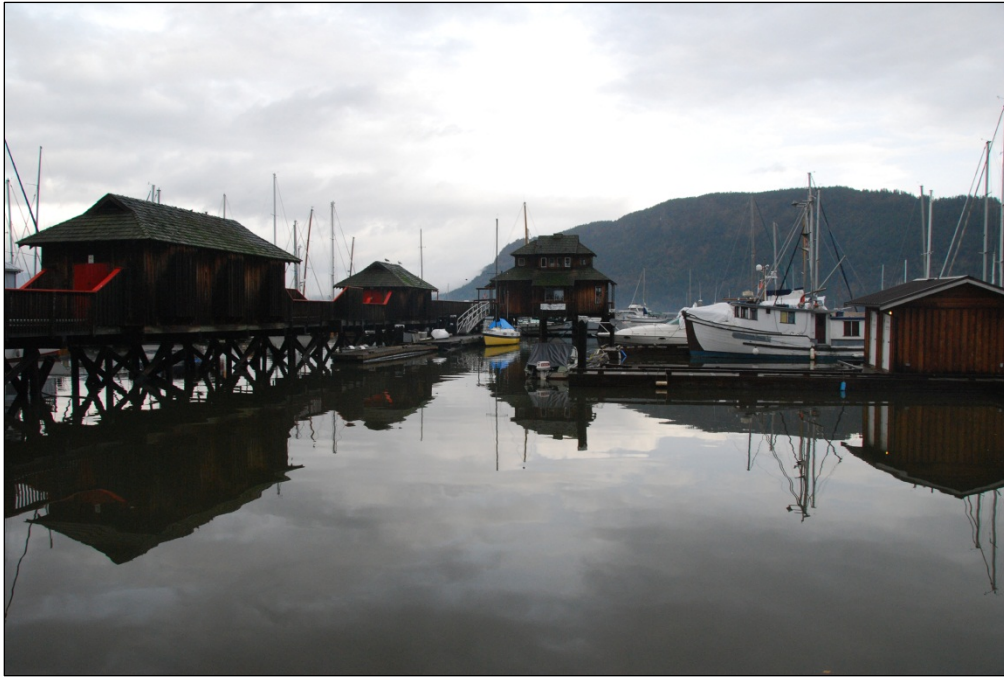
Photo 3: Pile supported structure: Wooden Boat Society
