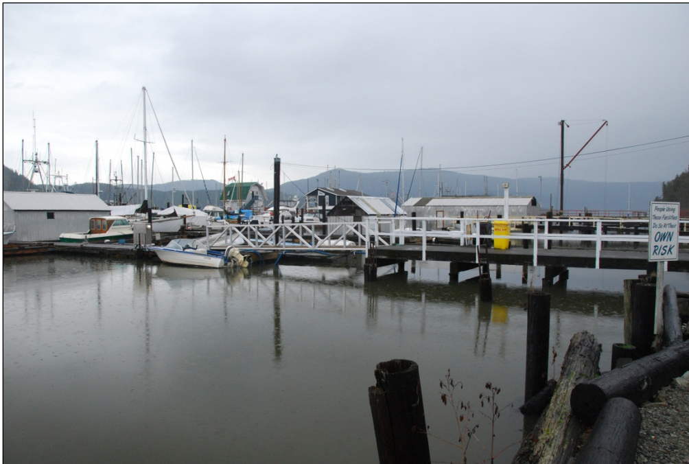
Photo 8: Pile supported walkway and boatsheds
